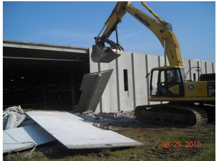
Removal of the concrete wall panels.
